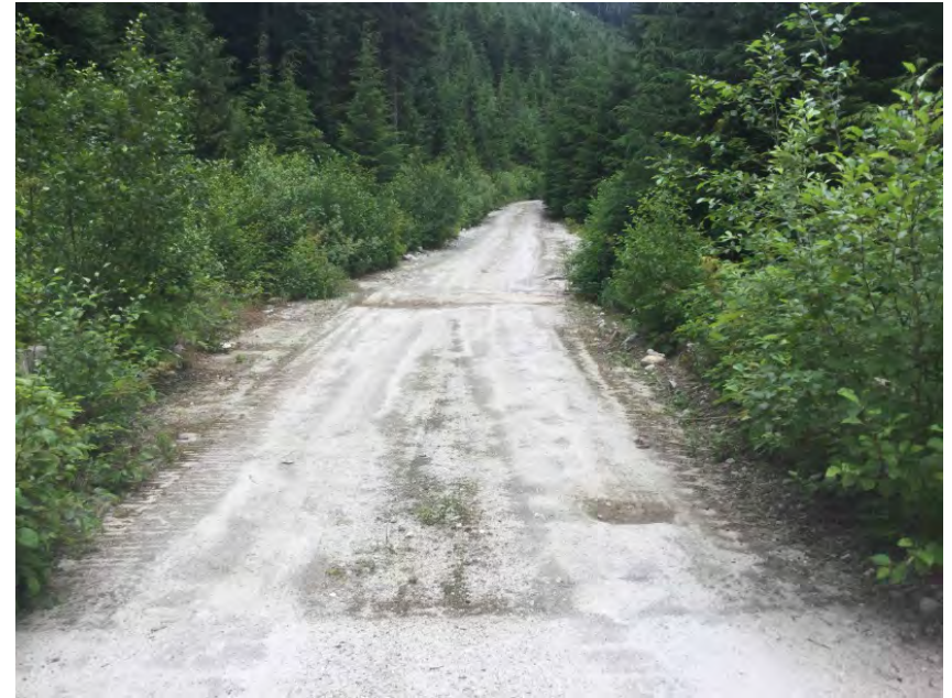
Left Approach Facing Away From Bridge
