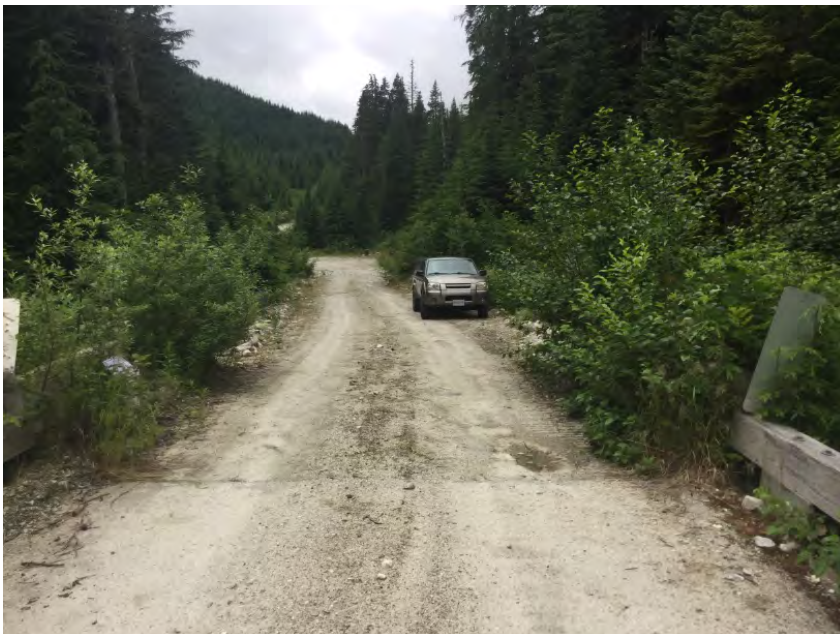
Right Approach Facing Away From Bridge
