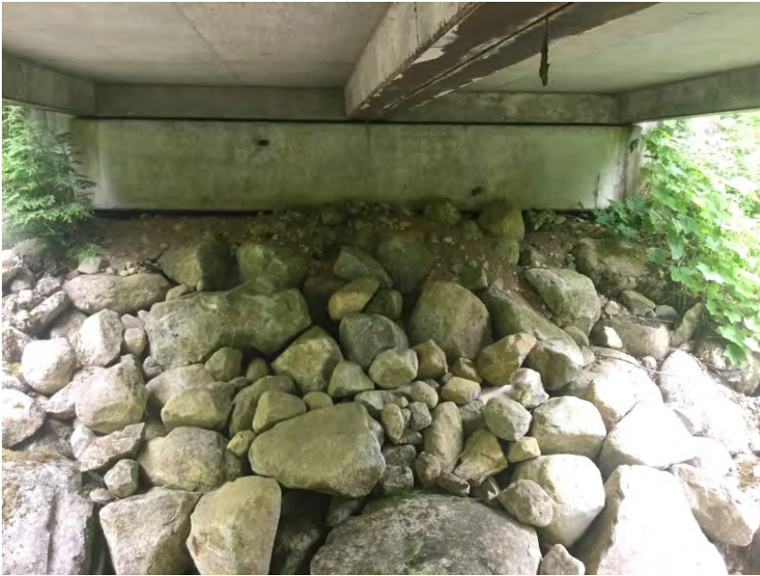
Left Bank Abutment
