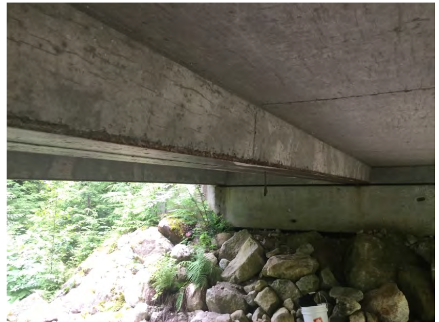
Compo Girder with Monolithic Deck
