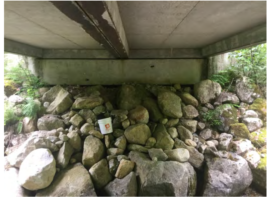
Right Bank Abutment
