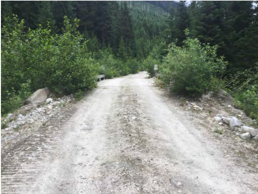
Right Approach Facing Bridge
